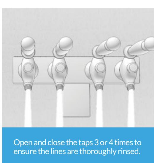
Open and close the taps 3 or 4 times to ensure the lines are thoroughly rinsed.
